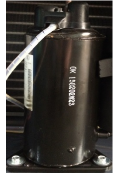
REFRIGERANT (FREON) COMPRESSOR HERMETICALLY SEALED REFRIGERANT COMPRESSOR EFFECTIVELY ELIMINATE REFRIGERANT FROM LEAKING
